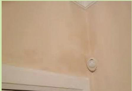
Penetrating damp shows as a wet patch and will not have any mould growth
