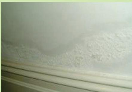
Rising damp is affecting the paint finish causing it to bubble.
