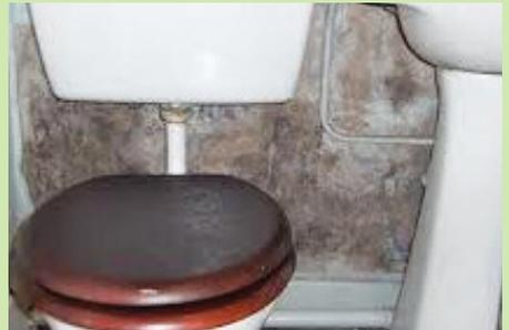
Condensation is the main cause of black mould. More than half the homes in the UK suffer some condensation problems.
