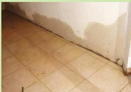
Rising damp shows as a water mark rising up the wall from under the floor.
