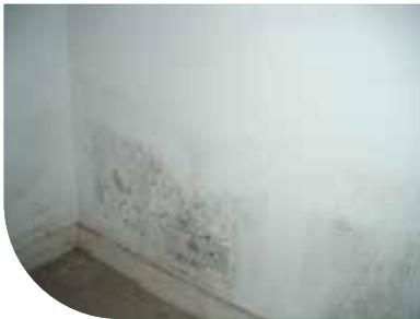
High levels of moisture in the air in one part of the building (such as within bathrooms and kitchens) can result in condensation occurring in another parts of the building as the moisture will pass to the colder parts of the house.
